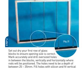
Panel anchors can be used as an alternative to drilling oversized holes and are an ideal alternative to drilling holes if the opening is a metal box section or steel I & H beam etc.
