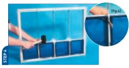
Fit first block and tamp down gently, fit second block and repeat. Ensure there is enough mortar between the blocks and the base to create sufficient adhesion. compact the vertical mortar joint using a wooden instrument. (fig.4) Note: Spacer pegs are not necessarily required between base and first row of blocks. When using spacers at the base or up the side jambs cut the legs of the cross spacer pegs to form at shape.
