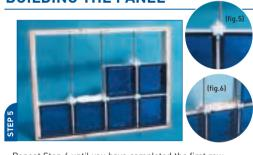
Repeat Step 4 until you have completed the first row. Insert spacer pegs in between blocks, this prevents steel rods from touching glass, assists with accuracy of vertical & horizontal joints whilst preventing mortar squeeze, enabling more courses to be constructed. (fig.5).
