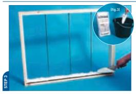
Mix Colmef Vetromix glass block mortar following instructions on reverse of bag (fig.3). The mix should be a semi dry consistency (Slump 1 or less). Lay down a bed of mortar
