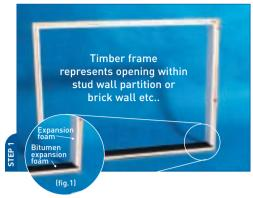
Calculate the correct opening size. Make sure the opening is square and perpendicular. Lay bitumen expansion material along base of opening. Secure expansion foam to jambs and head. All four sides of the opening should now be covered in expansion material Bitumen is necessary on the base to take the weight of the glass block wall.
